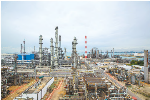
Shell Eastern Petroleum
